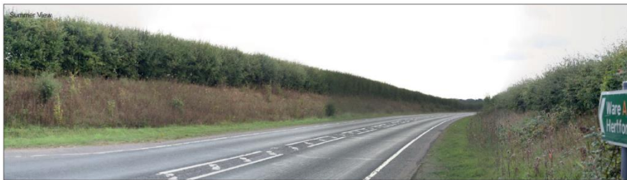
Figure 1 - A view of the single carriageway A602 in its rural setting
